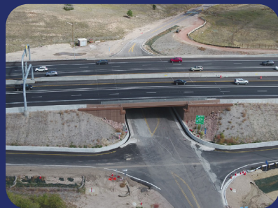
I-25 ML over County Road (2 structures)
