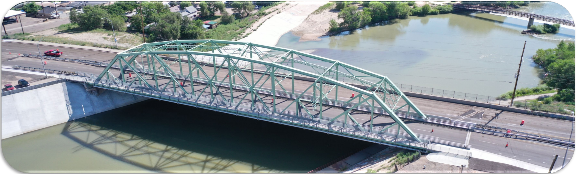
US 50 Business over Arkansas River - Historic Truss Bridge Rehabilitation
