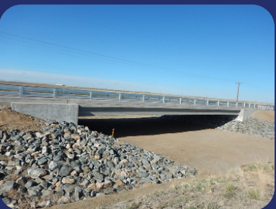
Eastern Plains Bridge Replacement Program - Package 1 (3 structures)
