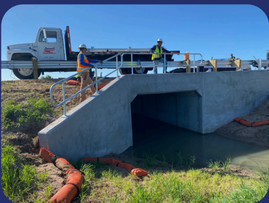
Eastern Plains Bridge Replacement Program - Package 2 (2 structures)
